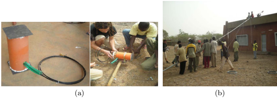
Fig. 4. (a) The antenna with a PVC radome ready to be installed; all the material is low-cost, recycled and locally available; (b) The set up of an antenna mast made by water pipes (third expedition, Jan. 2007)
