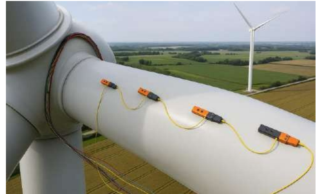
Figure 5: Field deployment of MEMS-FBG strain and acceleration sensors on wind turbine blades.
