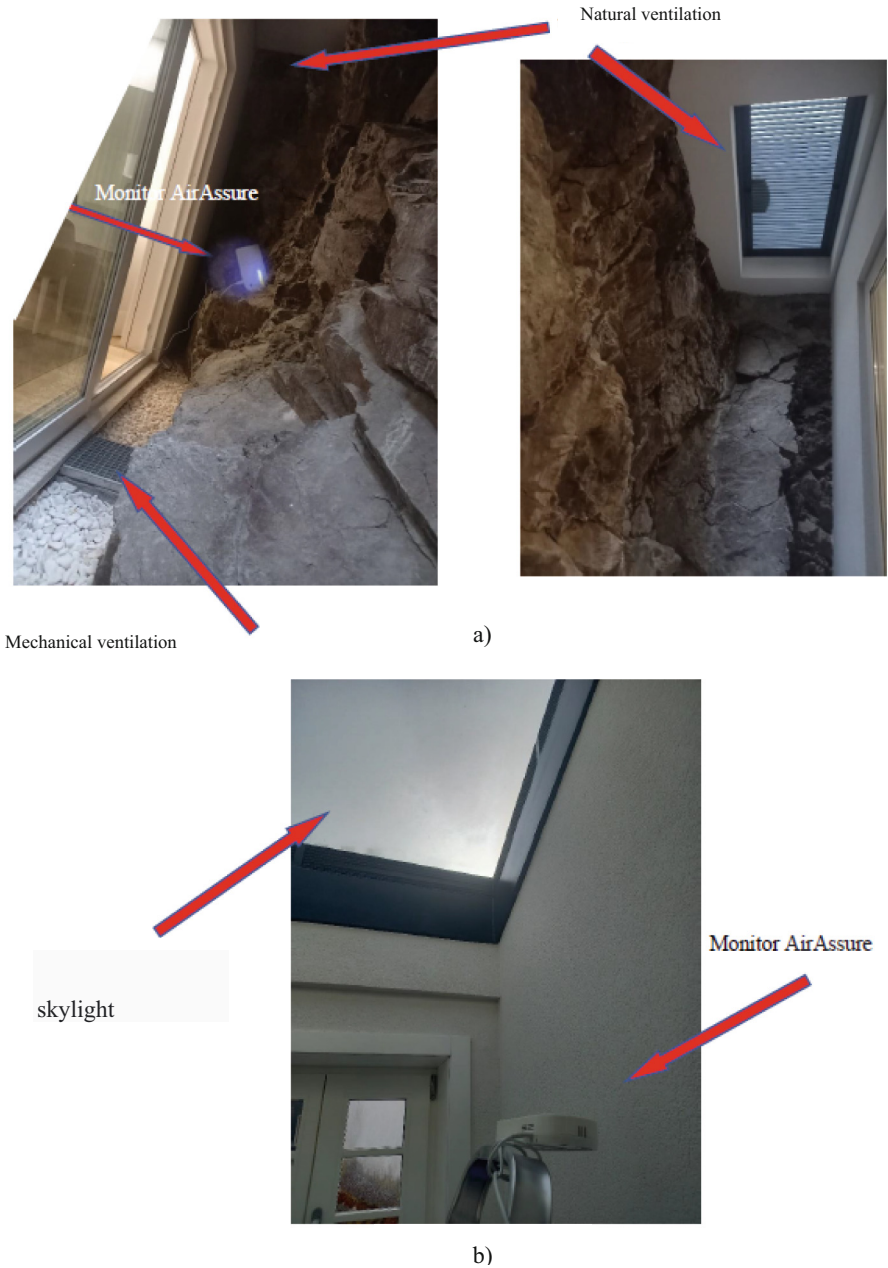
Fig. 4. Ventilation devices and sensors. a) Walls, b) Tower
