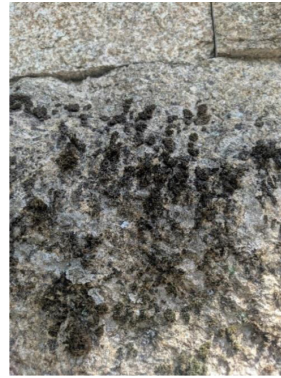
b) Details of the mosses in the façade
