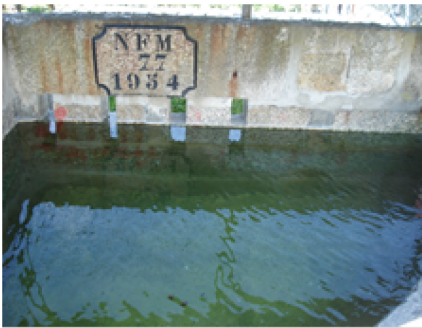
a) Washing tank
