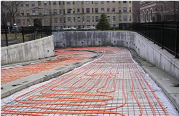
Fig. 1. Installation of solar road system collecting pipes
