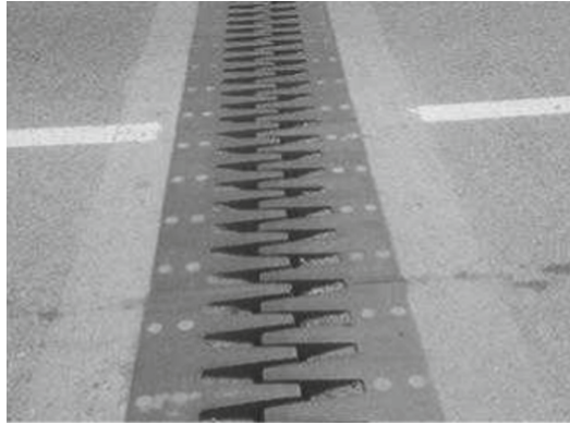
Fig. 1. Schematic diagram of highway bridge expansion joints
