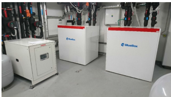
Fig. 2. Sources consist of heat pump for transformation heat and cold from earth and air. Left is combined heat pump of systems air-water and earth-water, middle and right is heat pump of system earth-water
