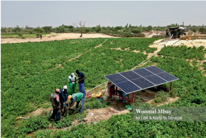
Fig. 3. Woomal Mbay System No. 1 used by the farmer, replacing the previous diesel-powered motor pump system in the background (source: Nadji.Bi Senegal Database).
