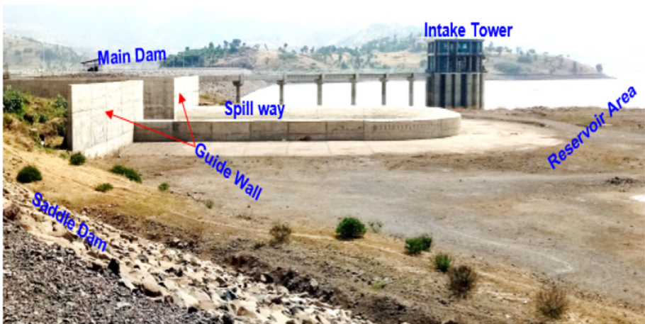
Fig. 14. Approach and control section of Ribb dam spillway
