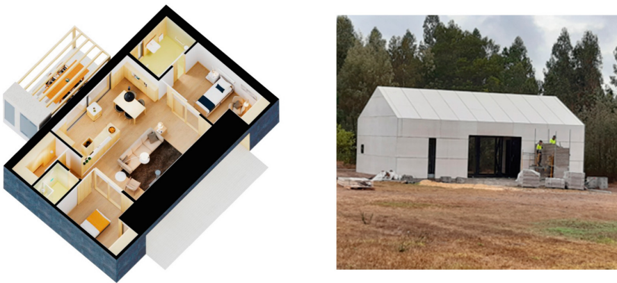
Fig. 1. On the left figure, the 3D model of the house of the “Health Home” project (“Casa da Saúde” in Portuguese) being built at Rovisco Pais Rehabilitation Center in Portugal ( https://www.roviscopais.pt ). The house consists of a large and central living room connected to the kitchen, a main bedroom with private WC (right side in the left figure) and a guest room and WC (left side). In the right figure, the construction of the house.
