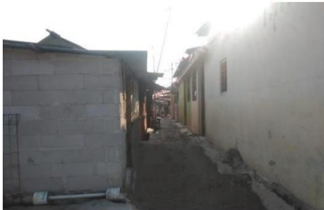
Fig. 3. Condition of House in Location
