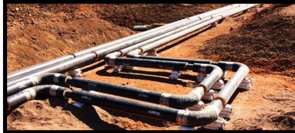
Fig. 1. Expansion loops in piping systems [2].
