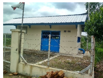
Fig 2. Irrigation source PWS
