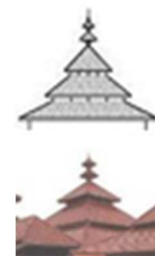
Figure 19. The tajug roof of Banten Great Mosque (five-tiered pyramidal type)
