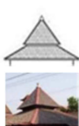
Figure 17. The tajug roof of Panjunan Great Mosque (two-tiered pyramidal type)
