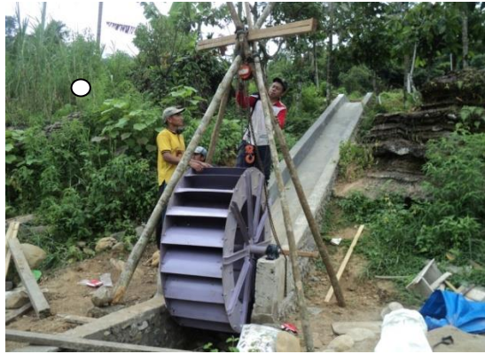
Fig. 7. Installation of the W2KDS on the ground
