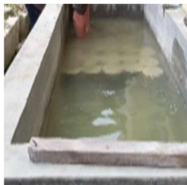
Fig 4 Concrete curing
