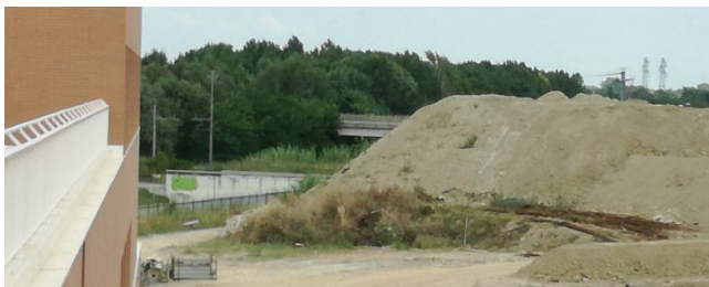
Figure 3: The artificial hill created to protect the building from pollution coming from the railroad and the highway.
