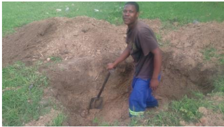
Fig. 4. Digging trial pits for geotechnical tests.
