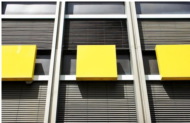
Figure 3. External shading system [18]
