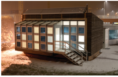
Figure 1. The Connected Sustainable Home in Trento.
