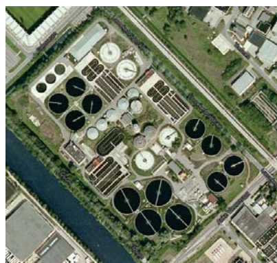
Figure 1: An eagle view picture of the sewage treatment facility in Enschede, the Netherlands. The picture is retrieved using Google Maps.
