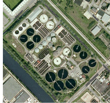
Figure 1: An eagle view picture of the sewage treatment facility in Enschede, the Netherlands. The picture is retrieved using Google Maps.
